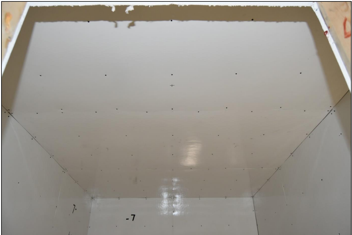
Figure A-2. Pretest View of Ceiling.
