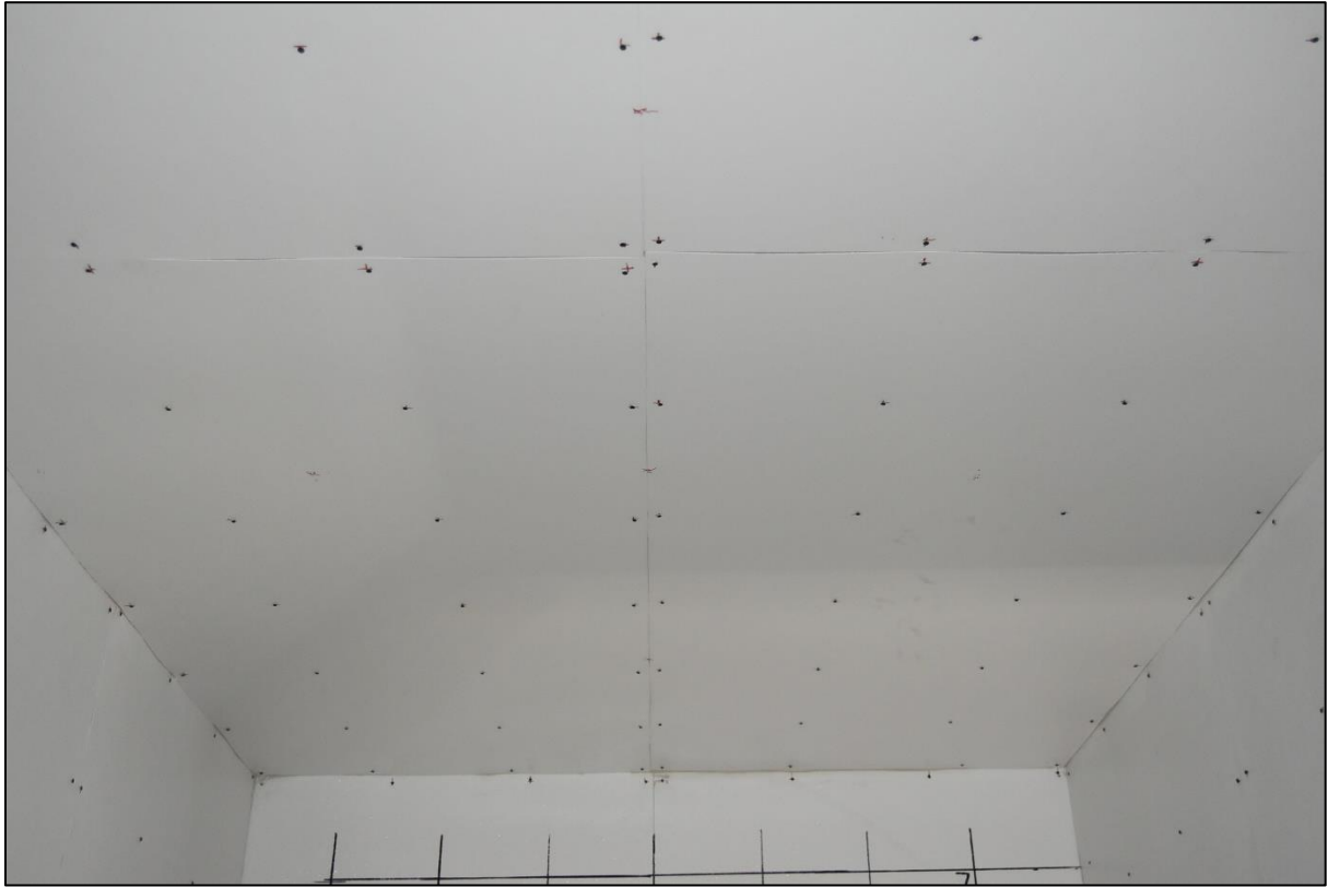
Figure A-3. Pre-Test View of Ceiling.
