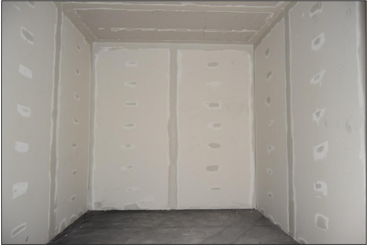
Figure A-1. Room Construction. Gypsum prior to Sample Installation.
