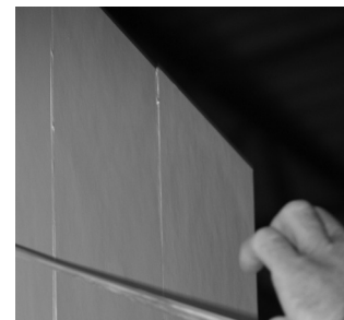
FIGURE 20: REMOVING PAINTER'S TAPE
