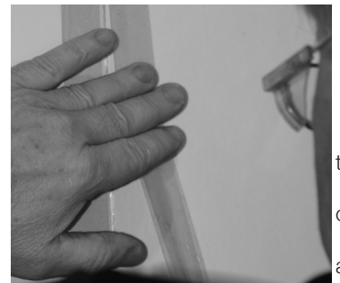
FIGURE 16: APPLYING THE PAINTER TAPE
