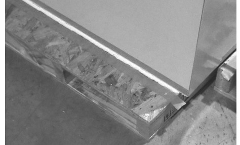
FIGURE 22: HORIZONTAL SEAM FILLED COMPLETELY WITH SEALANT
