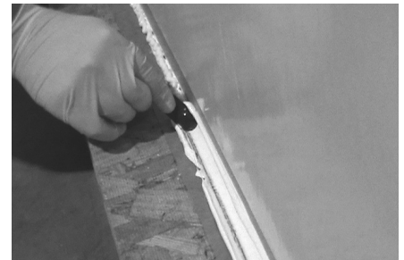
FIGURE 23: HORIZONTAL FINISH WITH ROUNDED CORNER
