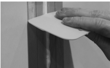
FIGURE 18: REMOVING EXCESS SEALANT
