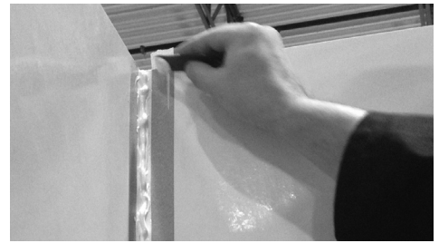
FIGURE 21: USING RADIAL SEAM FINISHER FOR ROUNDER CORNER JOINT
