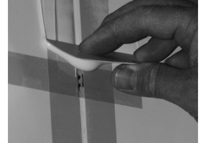
FIGURE 17: APPLYING THE PAINTER TAPE HORIZONTAL IN 3' SECTIONS
