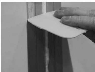
FIGURE 18: REMOVING EXCESS SEALANT
