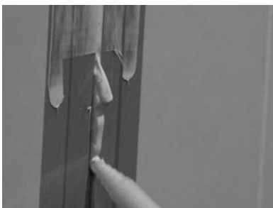
FIGURE 19: BUMP ADHESIVE IN TO PREVIOUS SECTION
