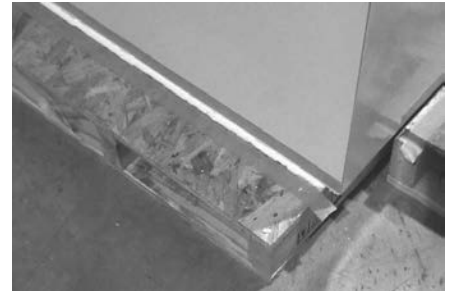
FIGURE 22: HORIZONTAL SEAM FILLED COMPLETELY WITH SEALANT
